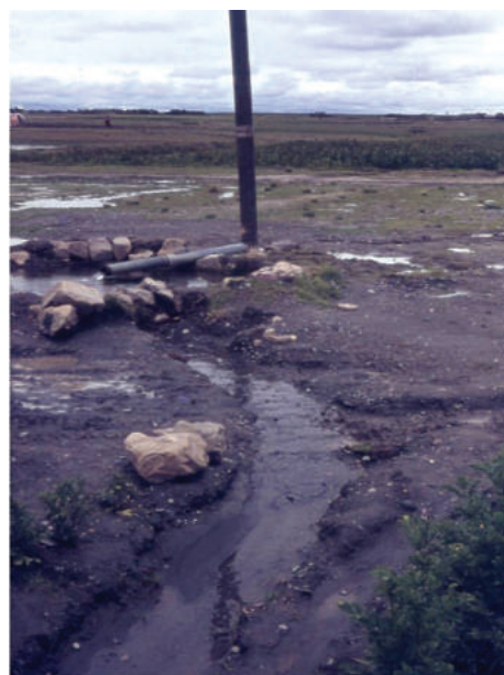
Figure 4.15 Artesian well on the Bolivian Altiplano. [Photo: Jac van der Gun]. The casing extends several metres above ground surface to ensure that no groundwater is spilt after the horizontal discharge pipe is closed.
